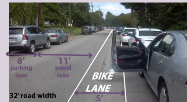
sub-standard space for door swing 8' parking lane
