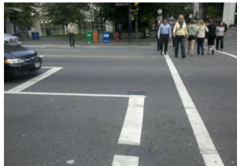
A staggered stop bar in Vancouver
