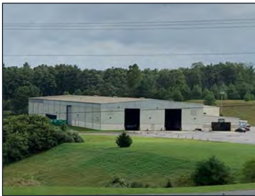
RCSWA Recycling Facility Exterior
