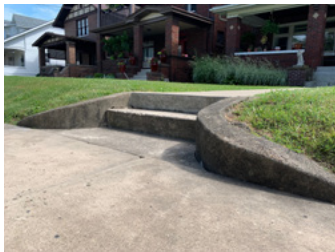
Above: Front yards in the district were designed with a gentle slope to the sidewalk and included a simple concrete curb. The curb above should be repaired. Replacement with a low block retaining wall is inappropriate. Below: The concrete curbing in the district was designed with rounded corners at the intersection of the sidewalk with driveways and stairs. This feature should be retained or restored whenever possible.
