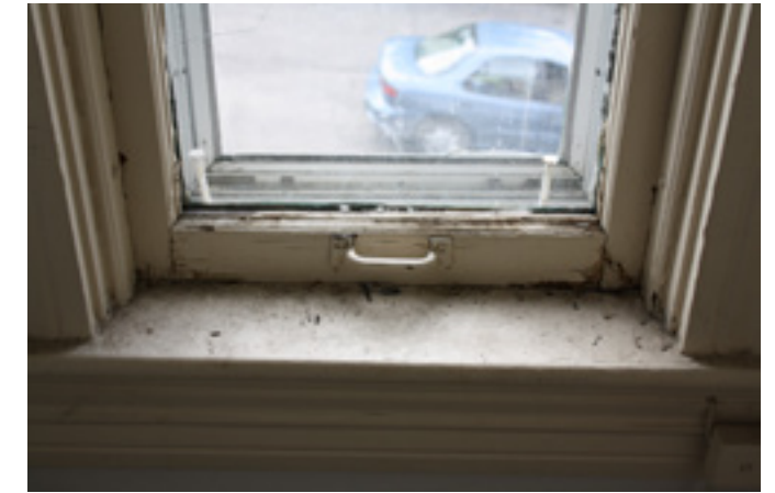
Upon brief visual inspection, a homeowner may conclude that this window is deteriorated beyond repair. But following the steps recommended here and in the National Park Service's Preservation Brief No. 9: The Repair of Historic Wooden Windows, the window was restored (below). Now it is weathertight, like new in appearance, and functional for many years to come.
