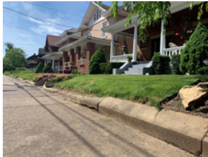
Above: Front yards in the district were designed with a gentle slope to the sidewalk and included a simple concrete curb. The curb above should be repaired. Replacement with a low block retaining wall is inappropriate. Below: The concrete curbing in the district was designed with rounded corners at the intersection of the sidewalk with driveways and stairs. This feature should be retained or restored whenever possible.
