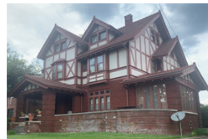
Masonry at the base of the character-defining front porch above is in need of cleaning by the gentlest means possible. Below, the mortar is missing at the base of this front porch. It is in need of repointing.
