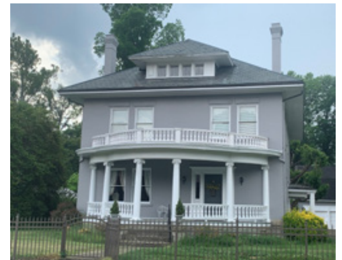
Below: Balustrades on this structure help to define its character. When the second story balusters fell into disrepair, the homeowner identified a contractor who was able to replicate their design in his workshop.
