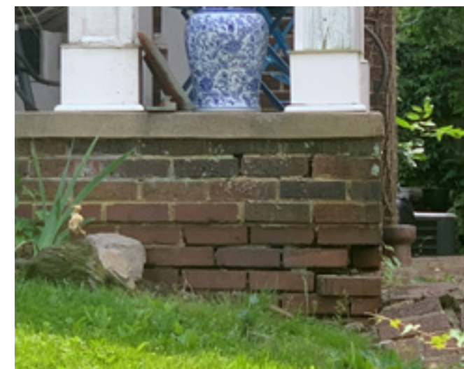
Masonry at the base of the character-defining front porch above is in need of cleaning by the gentlest means possible. Below, the mortar is missing at the base of this front porch. It is in need of repointing.
