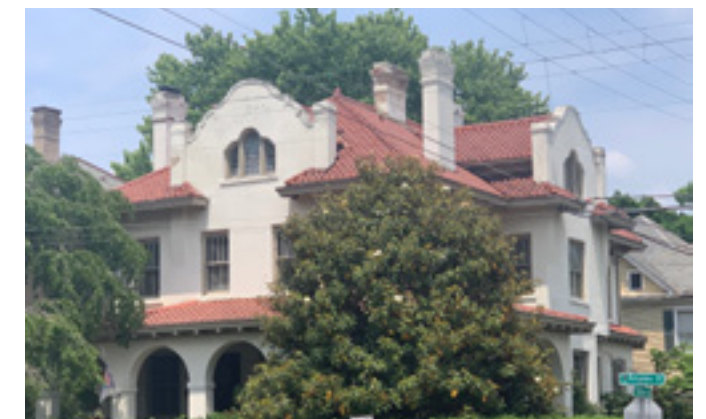
The Mission Revival features wide overhanging eaves, exposed rafters, gable or hipped roof of red tile, and Mission-shaped dormers or roof parapet.
