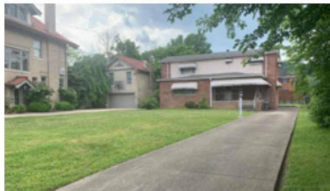
This structure is a departure from the character of the district in terms of its design and color palette. It is also set back on the rear of the lot, creating a gap in the rhythm and massing of Virginia Street.
