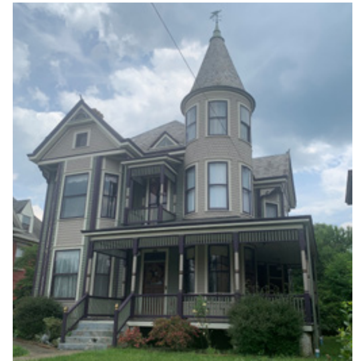
The Queen Anne style features a steep pitched roof with irregular shapes, a dominant front-facing gable, a hipped lower gable, a cross gable, decorative treatments on gabled ends, patterned shingles and spindle gable insets.
