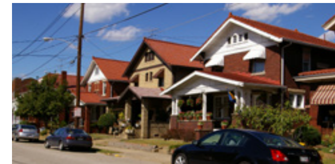
The repetition of architectural components of these structures creates the rhythm common in much of the East End Historic District.
