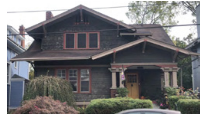
The Craftsman/Bungalow features low pitched gables, wide overhanging eaves, exposed rafter tails, and decorative brackets and corbels.
