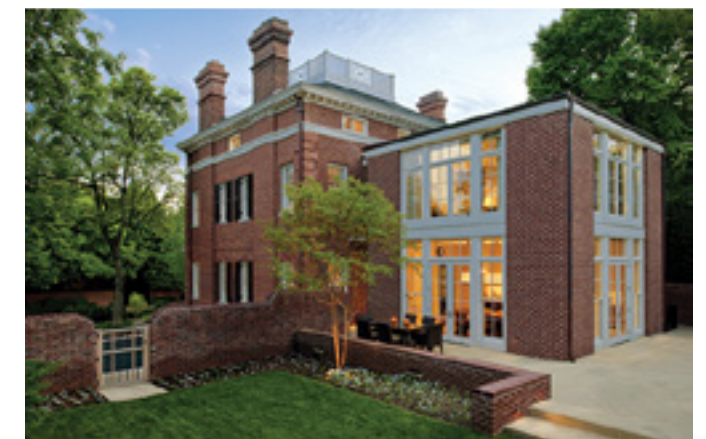
The addition in the image above, featured in the National Park Service's Preservation Brief on New Exterior Additions to Historic Buildings , retains the character and form of the original historic structure. It was placed on the rear of the building set back from the original structure, and it features similar a similar roof line and building materials.
